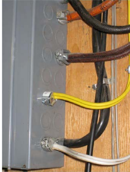
Figure 6: Example of cable clamping and grip devices. Image courtesy of University of Saskatchewan.
