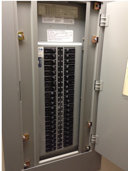
Figure 5: Example of a typical circuit breaker. Image courtesy of vaprotan, Flickr.
