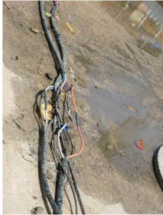
Figure 4: Frayed wires and power cables pose a significant significant electrical hazard. Image courtesy of marblegravy, Flickr.
