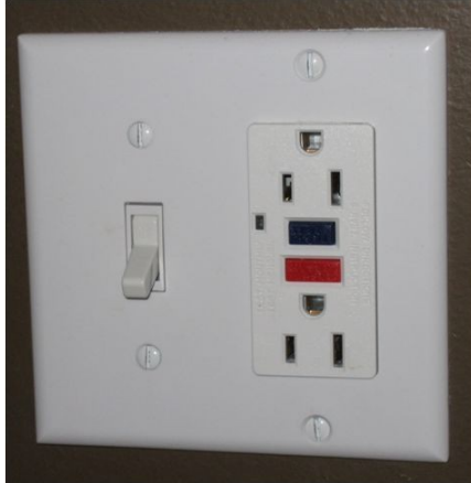
Figure 6: Example of ground fault circuit interrupter. Image courtesy of University of Saskatchewan.
