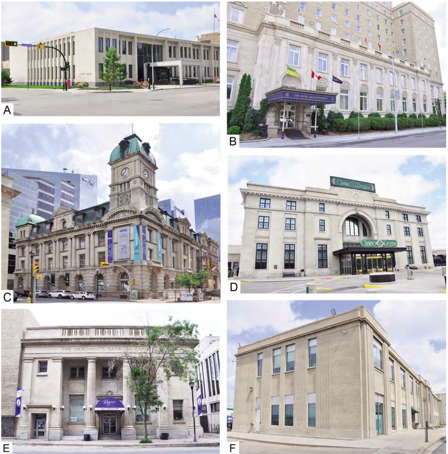
Figure 27. Examples of the range of building styles using Tyndall Stone, Regina. A. Courthouse (1961). Modernist style. B. Hotel Saskatchewan (1927). Neo-classical style. C. Post Office (1909). Beaux Arts style. D. Union Station (1911). Simplified Beaux Arts–Classical style. E. Merchants Bank (1911). Neo-classical style. F. CN/CP Telegraph Building (1932). Art Moderne style.
