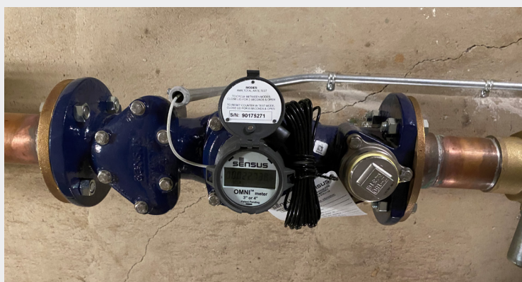
Installation of new water meter and water feed
